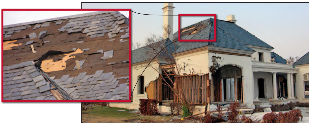
Figure 11-53. Damaged slate roof with nails that typically pulled out of the deck. Some of the slate broke and small portions remained nailed to the deck. Estimated wind speed: 130 mph. Hurricane Katrina (Mississippi, 2005)
